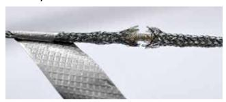
9. Smooth and seal the conductive tape to complete your splice.
