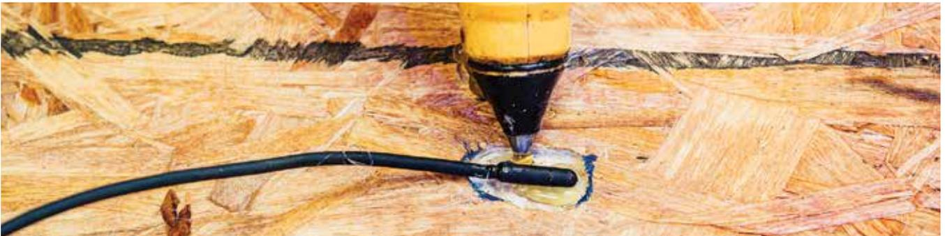
Figure 8. Secure the temperature sensor to the subfloor.
